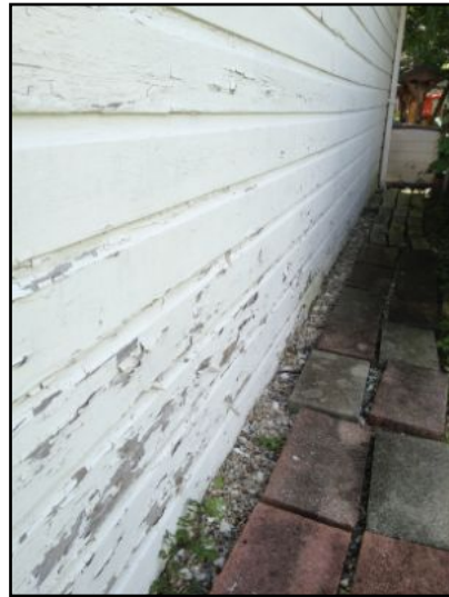
exterior walls of the garage could benefit from a new coat of paint
